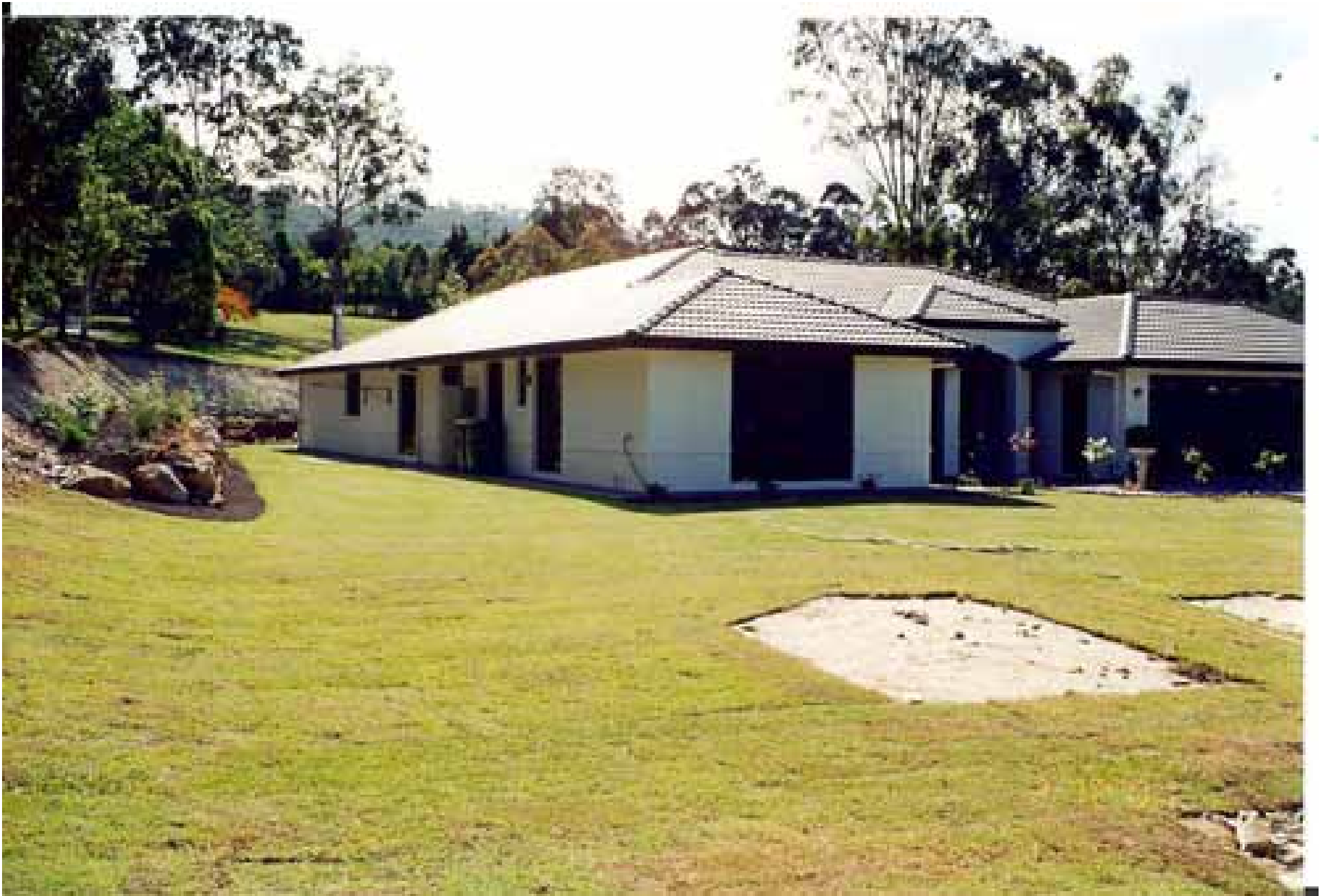
December 2001 - Grass is laid, the natives on the bank are growing and Angela comes up with a design solution' to hide the sewerage system
