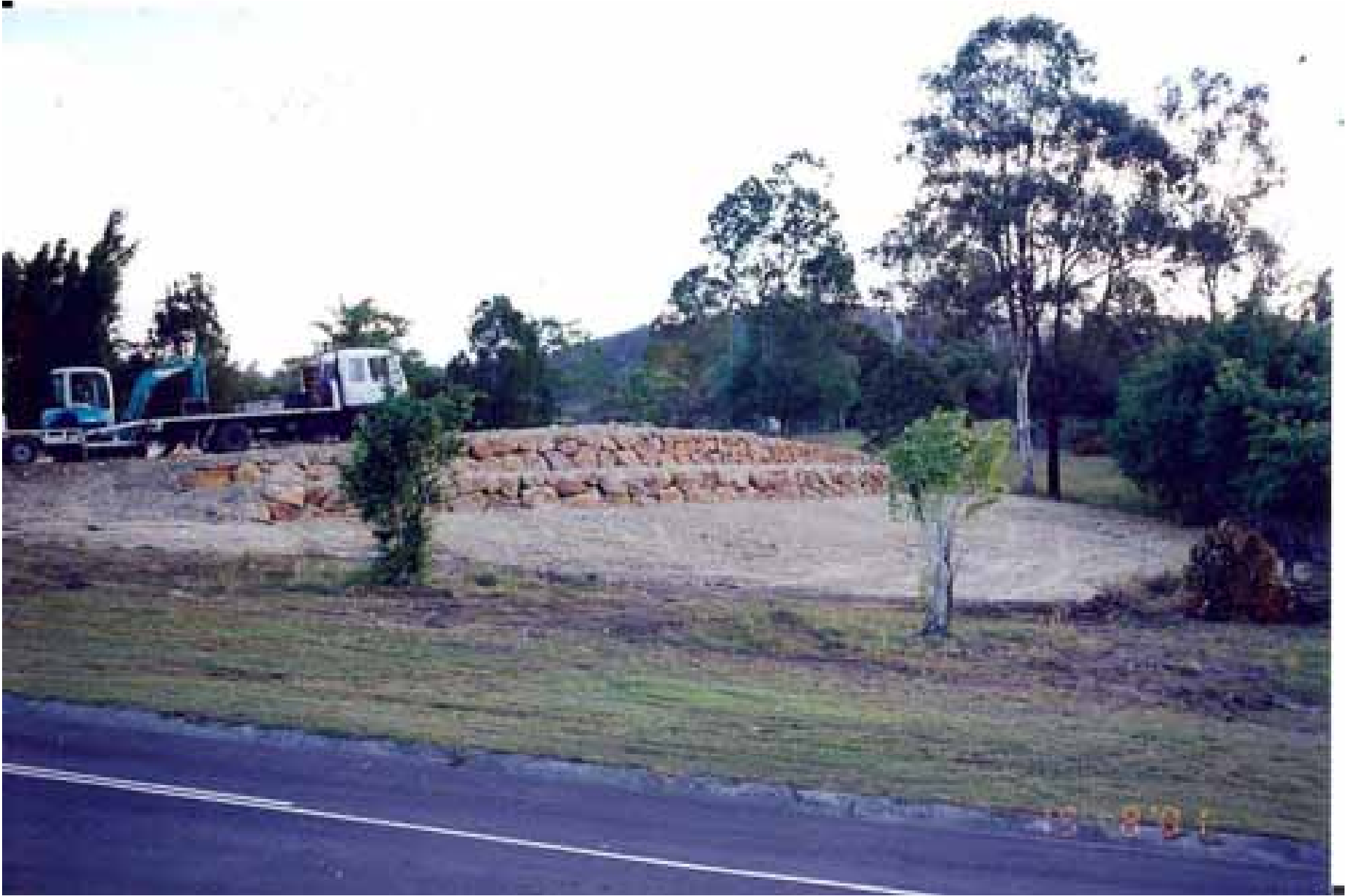
The retaining walls go in
