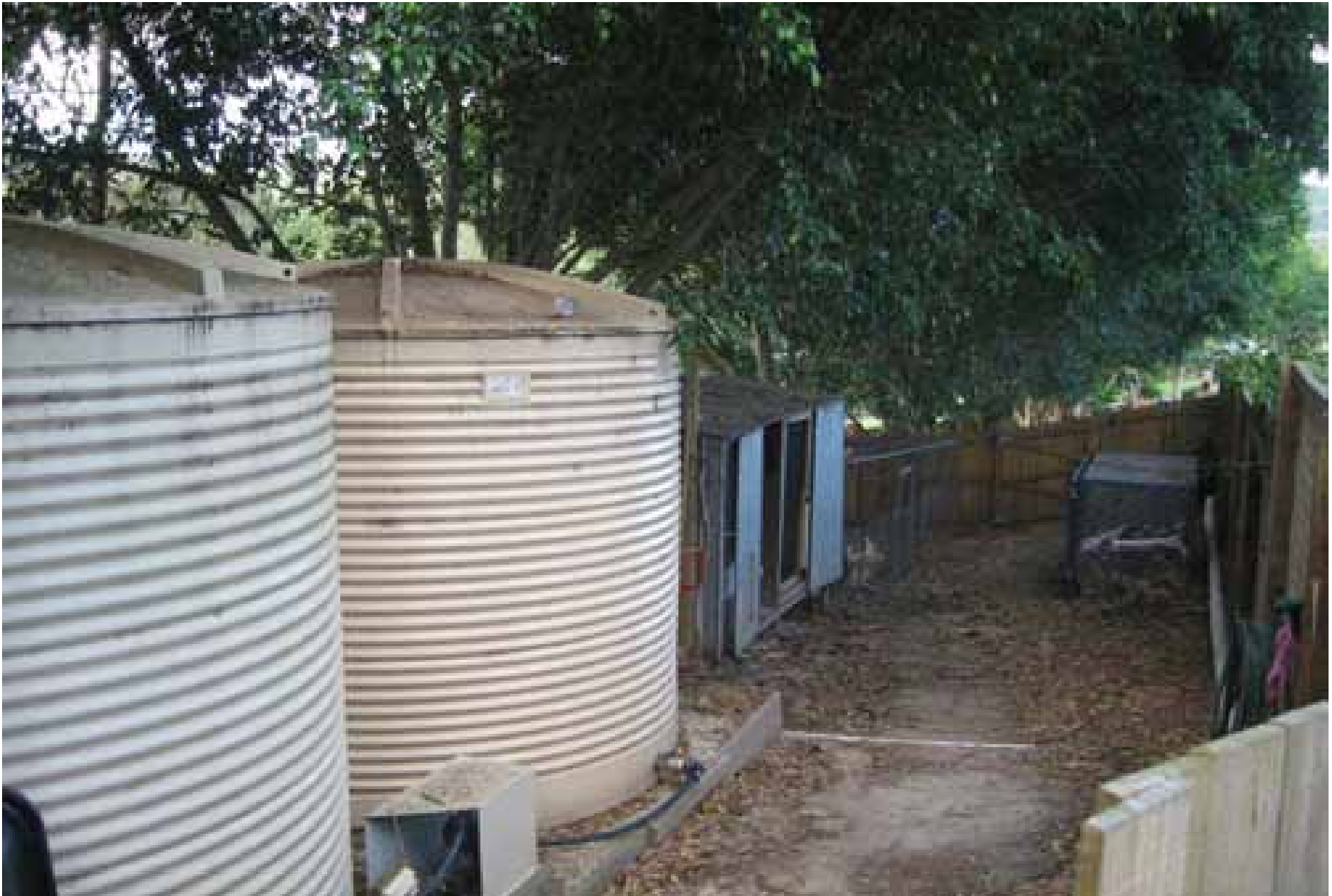
Two 12,000 Litre tanks ensure enough water for the plants Henhouse and compost bins in the background.
